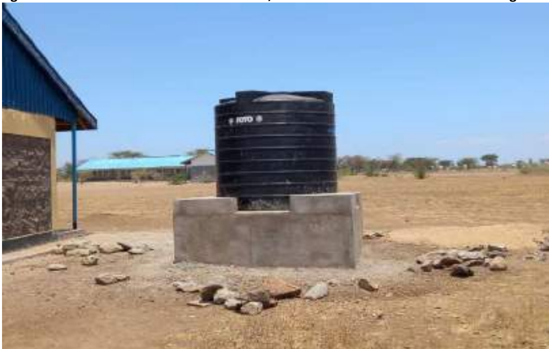
Figure 51. A Water on an Elevated Platform, Children on Wheelchairs have Challenges of Access
