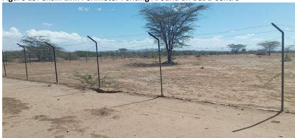
Figure 15. Chain Link Perimeter Fencing Around an ECDE Centre
