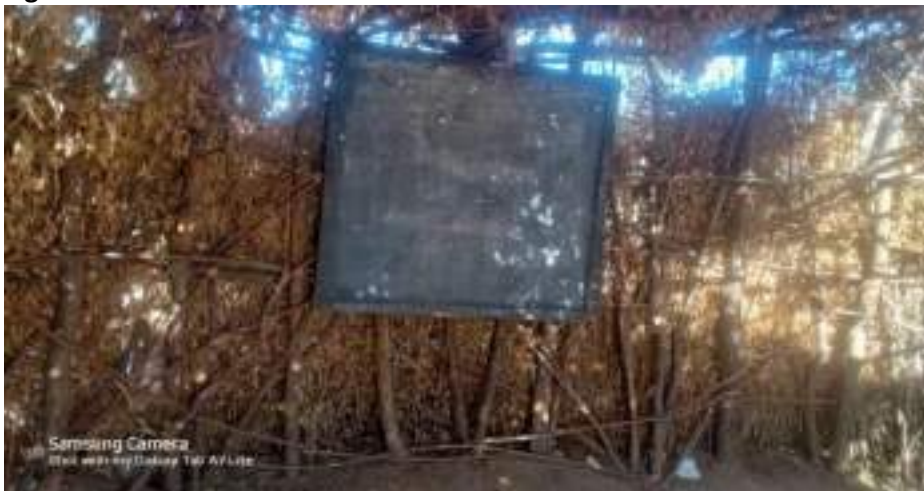
Figure 22 a. An ECDE Classroom with Thatched Walls and Roof
