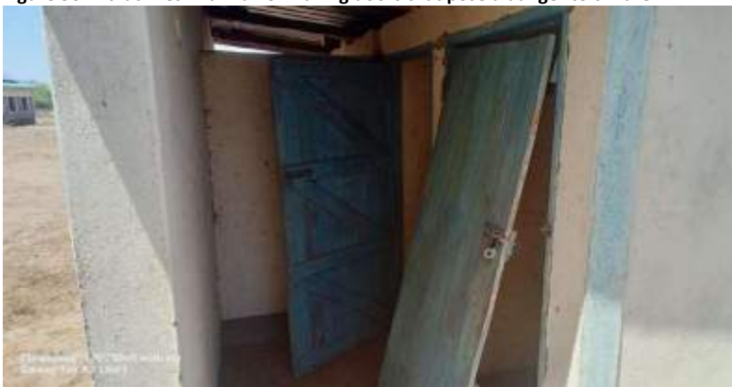
Figure 56. Pit latrines with narrow falling doors that pose a danger to children
