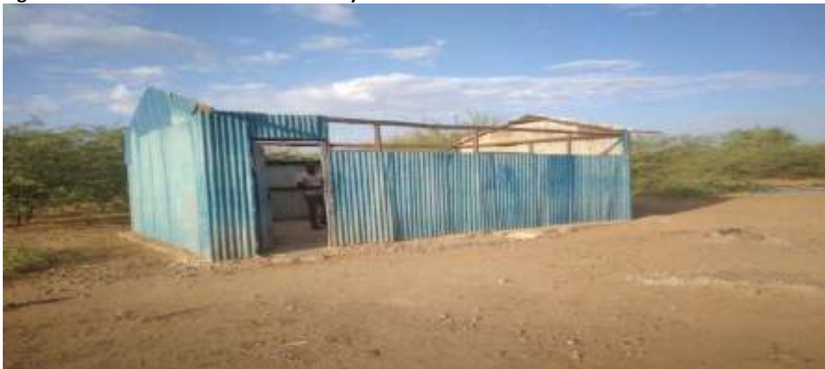
Figure 9 a. An ECDE Centre constructed by Iron sheets
