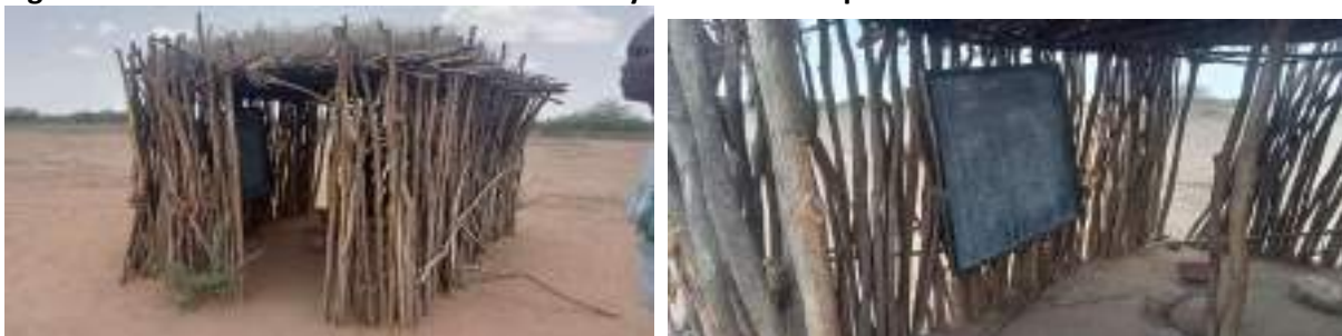
Figure 9C: A classroom constructed with locally available tree poles.
